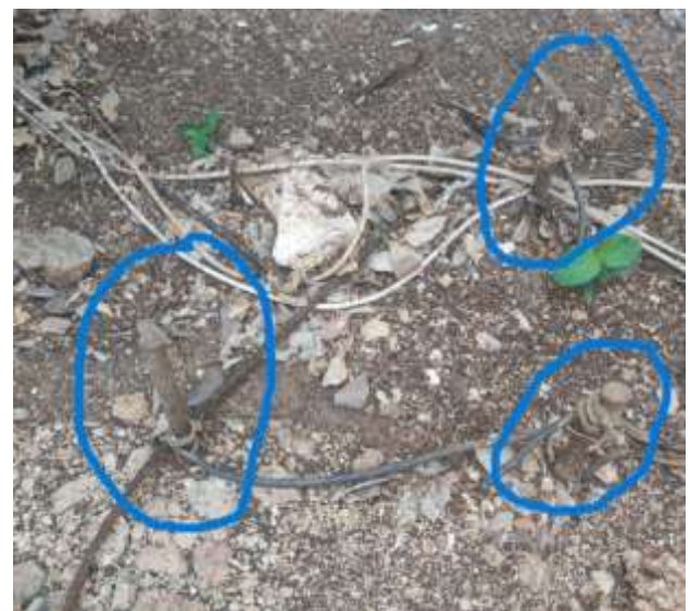
Figure 1 Delta grounding system Own Elaboration
