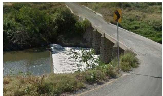
Figure 6 Bridge Source: (Google Earth) Simulations
