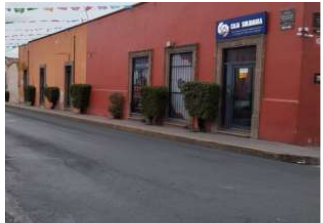
Figure 7 Facades of Huichapan Source: Project archive, 2023
