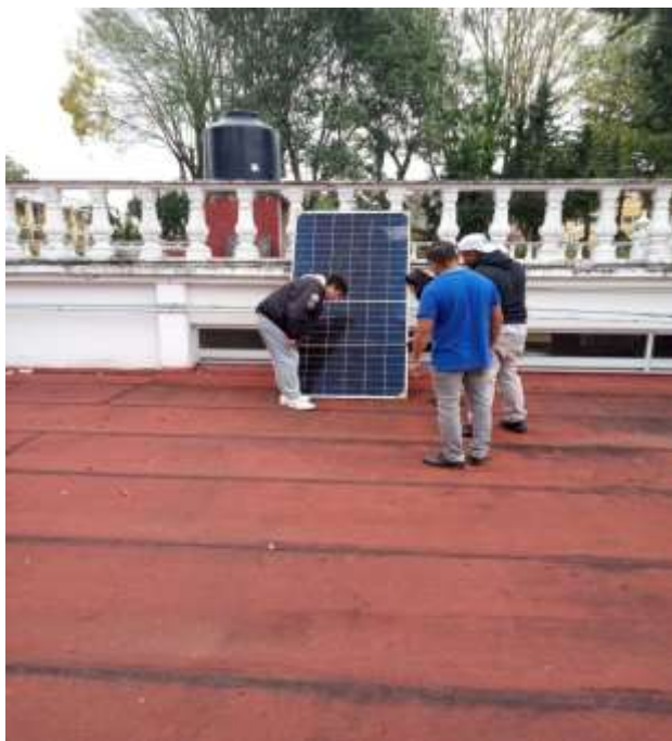
Figure 4 Solar Panel Installation
