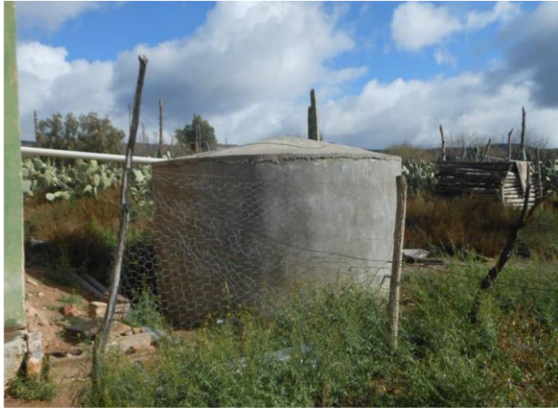
Figure 7 Storage tank type
