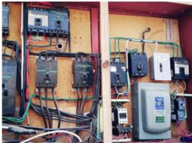
Figure 6 Load Center Source: Own Elaboration
