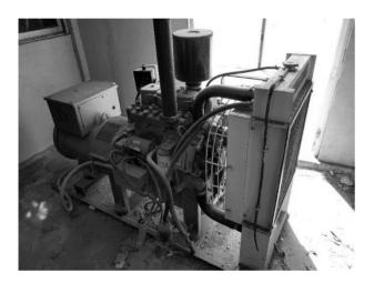
**Figure 3** Emergency electric generator of the clinic, operated with diesel *Source: Own elaboration*
